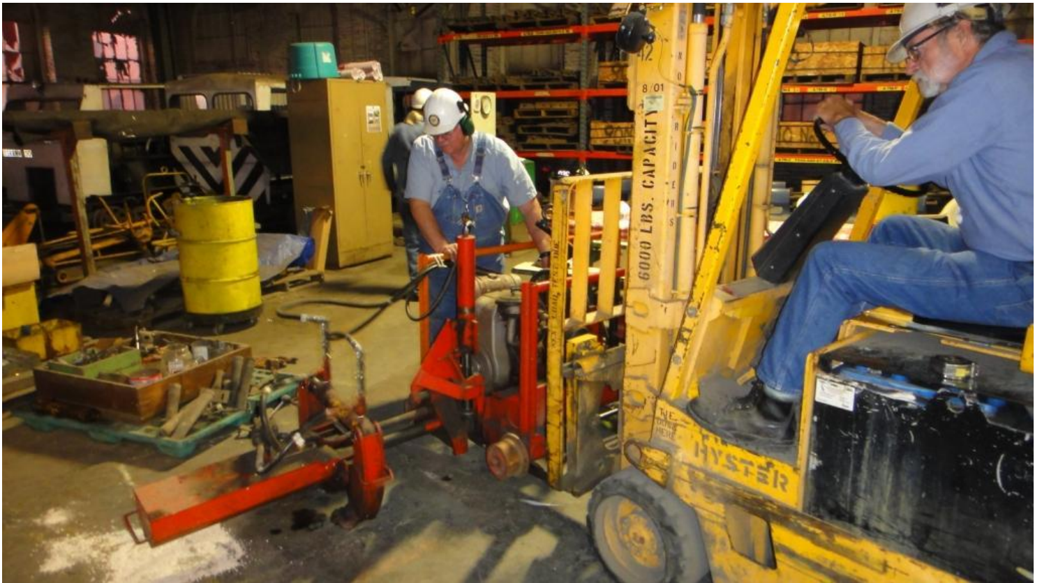
Chris testing the new squeeze-cylinder on the secondary section-gang machine that Frank and Josh installed last week
