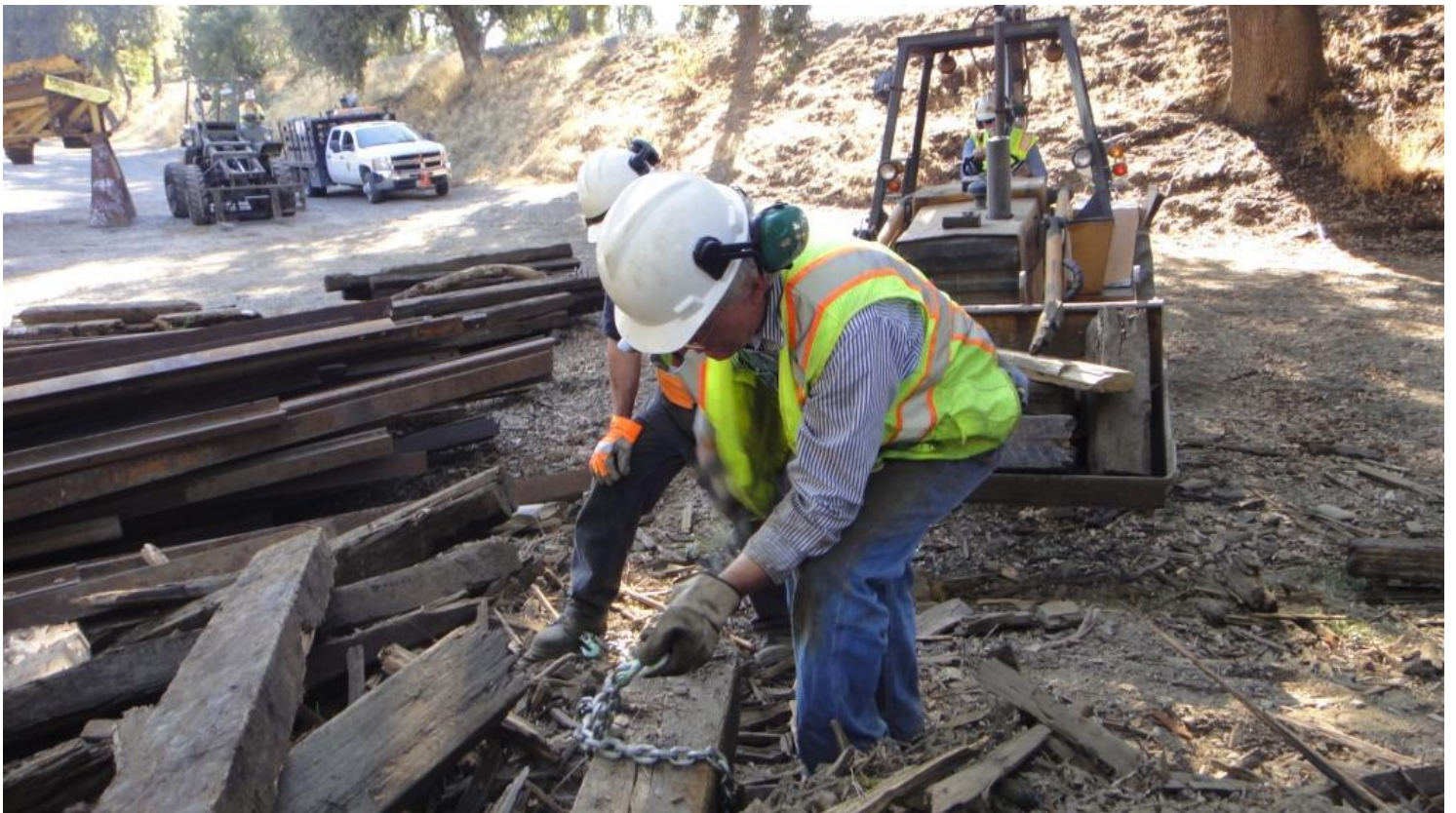
Steve and Fred attach chains to several ties which Alan will pull out with the back-hoe
