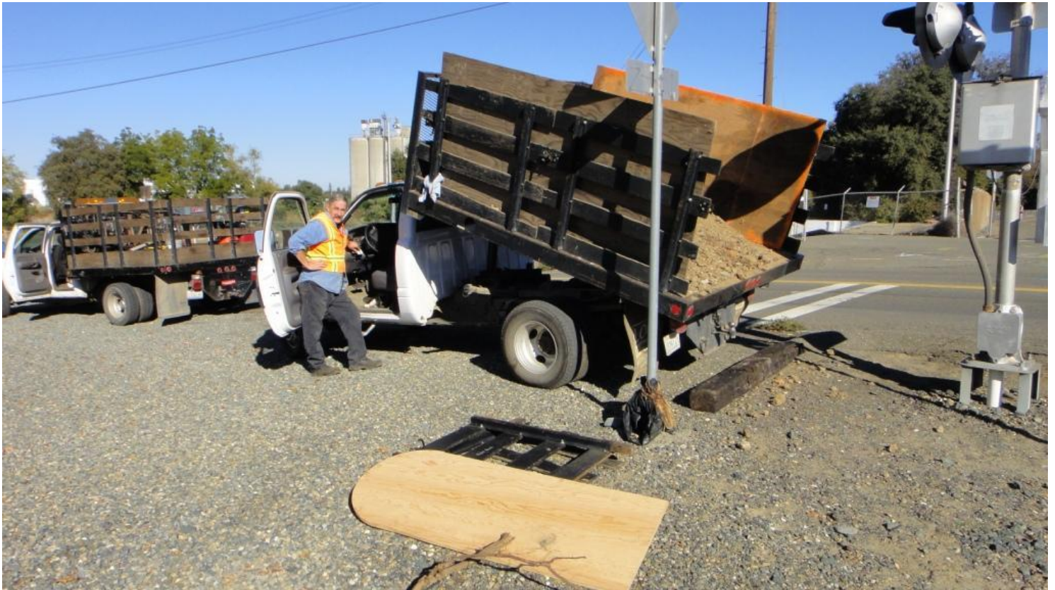
Fred operating the lift mechanism of the dump-bed to lay fill dirt around the crossing gate tower at Broadway
