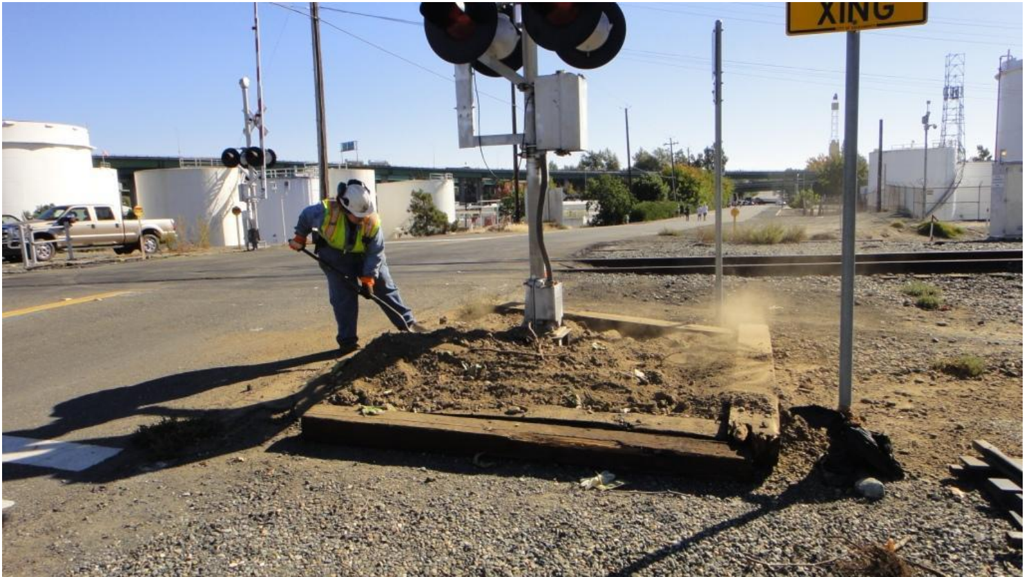
Talk about a lone worker – Heather spreading the dirt to make an even surface
