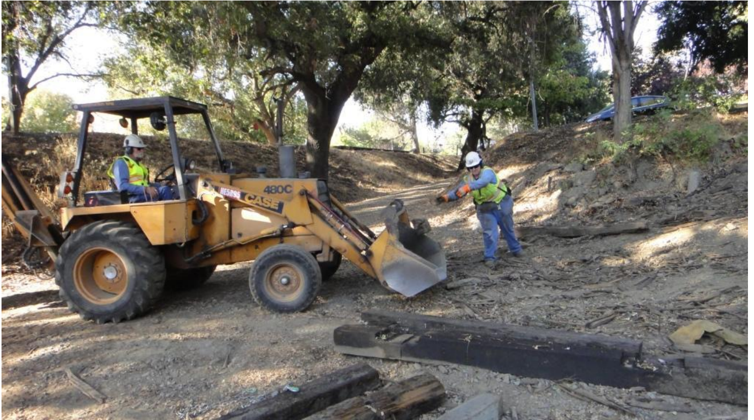
Heather tosses a broken tie into the back-hoe bucket
