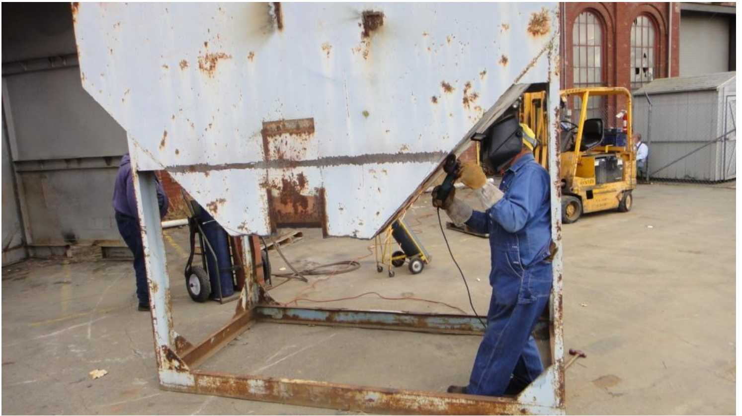
Cliff grinding away old paint and rust as he prepares to cut the side-dump "shoot" off the rock hopper that we're converting to a center-dump ballast hopper
