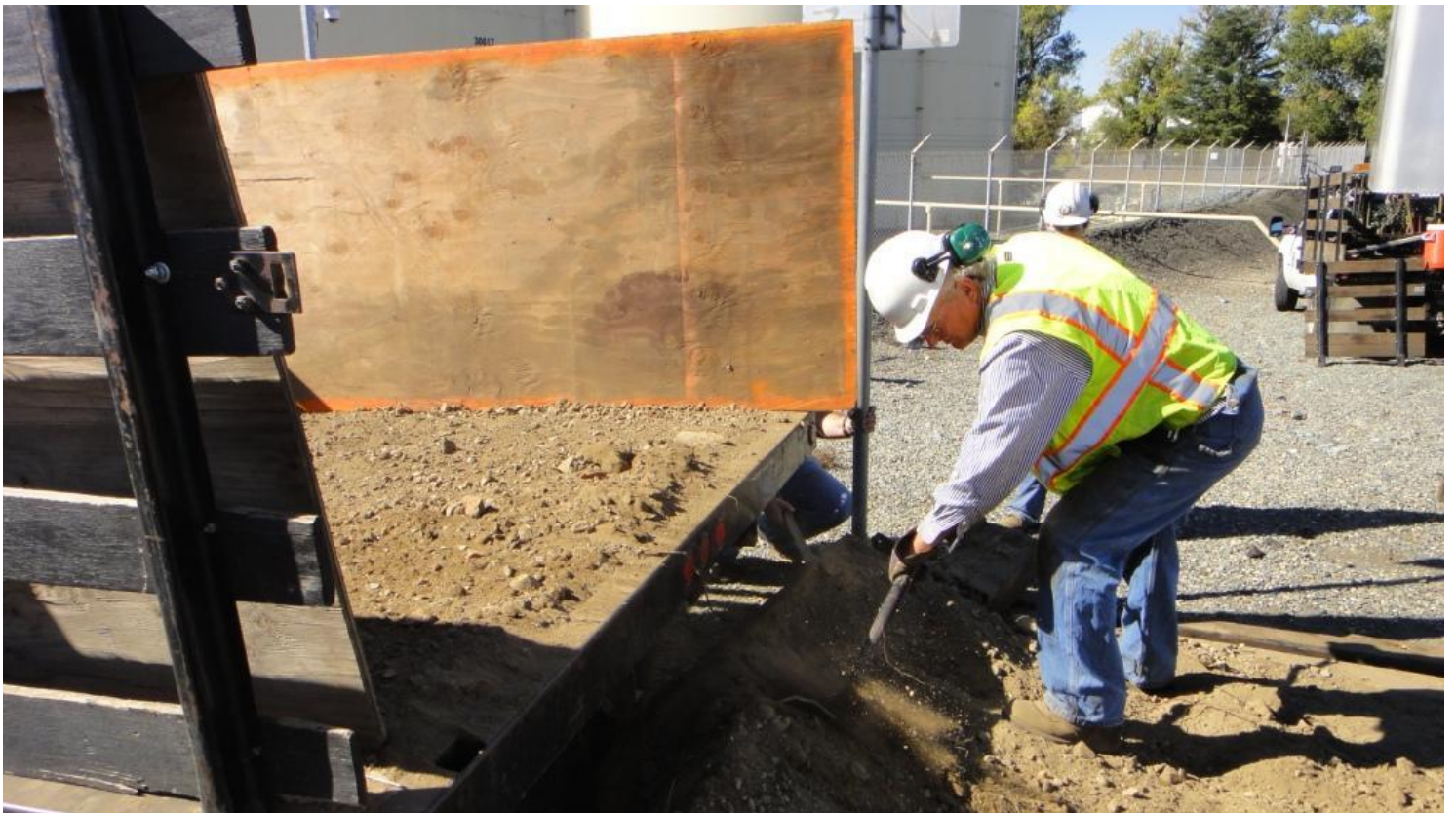
Steve handling the second load of dirt
