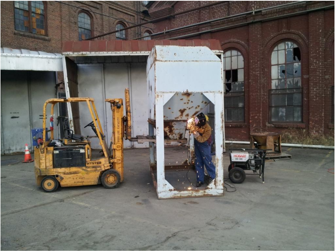
Cliff welding the reversed dump-shoot on the new center dump ballast hopper
